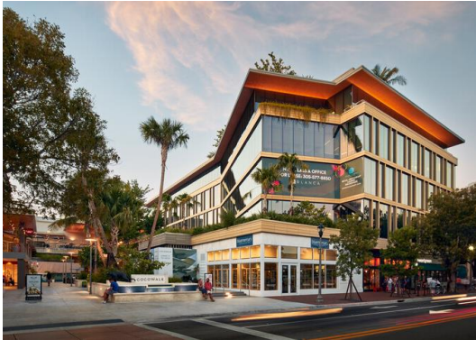
COCOWALK | Coconut Grove, FL 106,000 office/retail building $6 million remaining spend Retail 100% leased, office 98% leased
