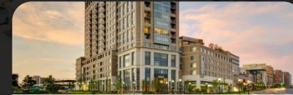
Pallas at Pike & Rose North Bethesda, MD 319 Residential Units | $125M
