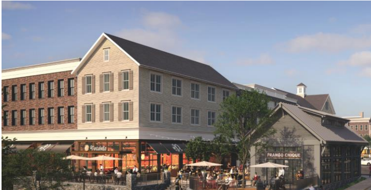
DARIEN COMMONS | Darien, CT 75,000 SF of new retail, 122 apartments $24 million remaining spend 2023 Anticipated Stabilization
