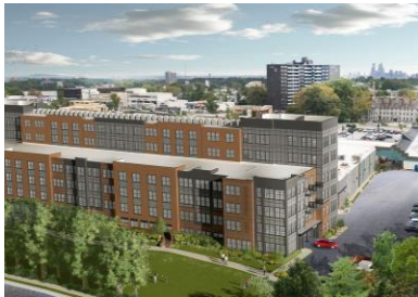
THE DELWYN – Bala Cynwyd, PA 87 residential units $2 million remaining spend Leasing commenced with move ins beginning late 2020
