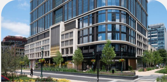
915 Meeting Street | North Bethesda, MD Mixed Use Expansion Projected Cost: $180 - $190 million Project ROI: 6% 91% committed 1
