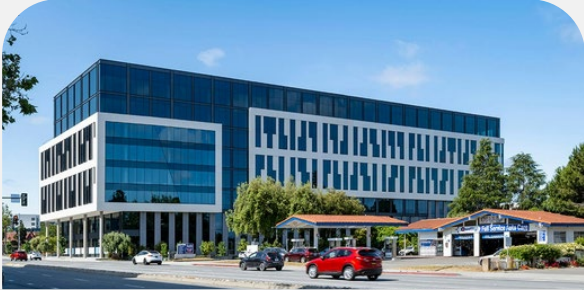
Santana West | San Jose, CA Mixed Use Expansion Projected Cost: $325-$335 million Project ROI: 5%-6% 82% committed 1
