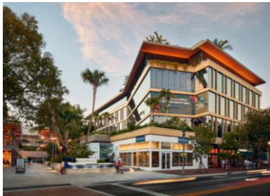
COCOWALK | Coconut Grove, FL 106,000 office/retail building $8 million remaining spend Retail 100% leased, office 98% leased
